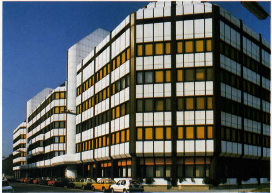
Construction of the new archive building in Vienna-Erdberg.
