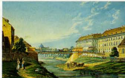
Water-colour painting by Ludwig Wülffinger of a chain bridge built in 1828 across the river Wien and linking the Viennese districts of Mariahilf, Margareten and Wieden.
